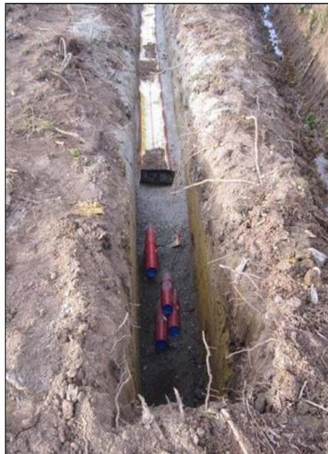
Plate 4-9 Typical Cable Trench View
