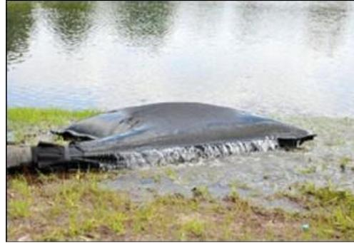
Plate 4-7 Silt bag under inspection
