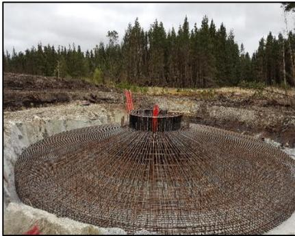
Plate 4-2 Turbine Base 'Anchor Cage'
