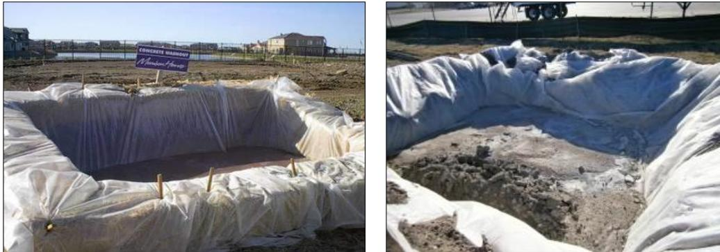
Plate 4-4 Concrete Washout Area
